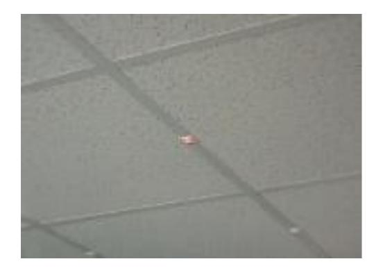
8. If the clip will be used, lift the ceiling tile and the halo tile and pull the clip into place on the rail, then push up the clip wires while lowering the ceiling tile until the clip is secured and the ceiling tile is in position. The arrow on the clip should point the ceiling tile with the HaloTile on top.
