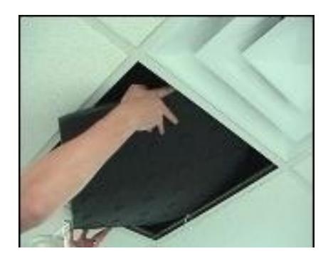
7. Now, place the HaloTile on top of the ceiling tile with the RED end of the white cable hanging out for the next Halotile. (unless this is the last HaloTile to be placed)
